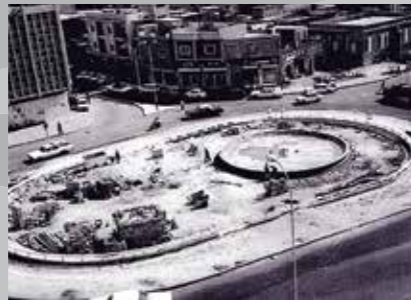
Arab Bank roundabout under construction
